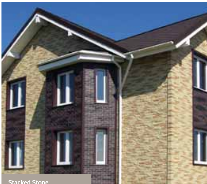
Stacked Stone, Hand-Laid Brick
